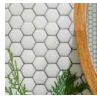
Junta gris // gray grouting.
